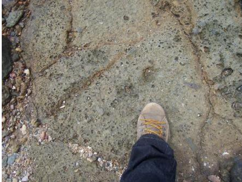
Photo 3 Close up of rock pavement.
